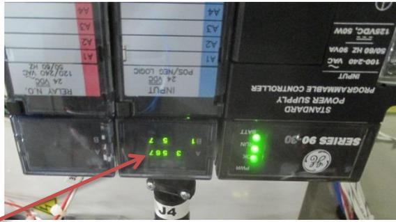
9. If the #A7 status indicator of the PLC input display is illuminated: rotate the pressure switch A adjustment screw to decrease the pressure using a 3/8" end wrench until the #A7 status lamp of the PLC goes out.
