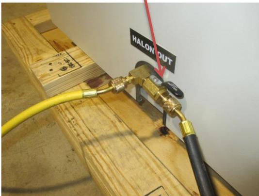
If the storage container DOES NOT CONTAIN AGENT: Open the vapor valve of the storage container: this will evacuate the container along with the plumbing connections at the same time.
