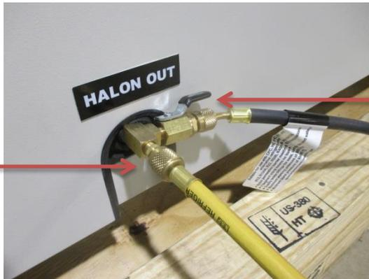
A hose connection from the Nitrogen Supply Evacuation Valve may be used to pressurize the plumbing in place of using a second source of nitrogen gas.
