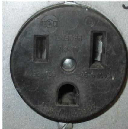
The mating receptacle for the plug is a USA NEMA type 6-50R 2-pole 3-wire ground receptacle, Hubble part number 9367 or equivalent.
