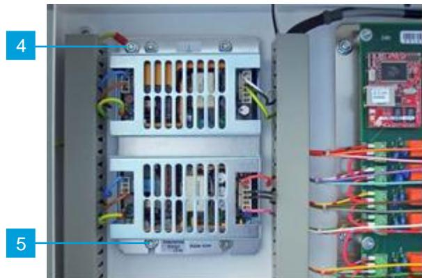
Fit the new power supply module complete with insert plate. Fit the shake-proof washers and securing nuts and tighten. Securely reconnect all cables previously disconnected.
