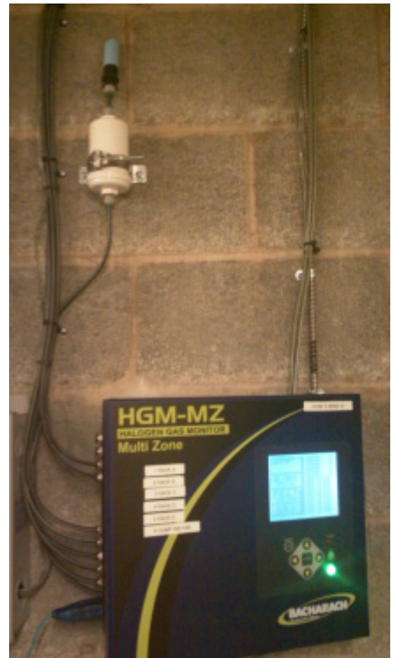
Figure 7. Indoor Filter Mounting Example
