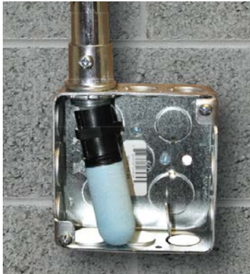
Figure 2. Best Practices: End of Line Filter for Dry Locations
